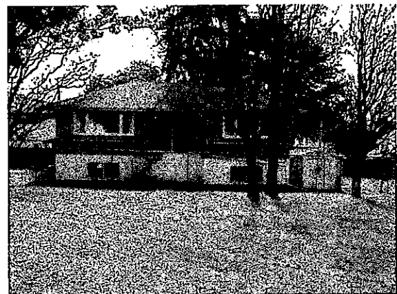
Figure 3. Existing dwelling unit
