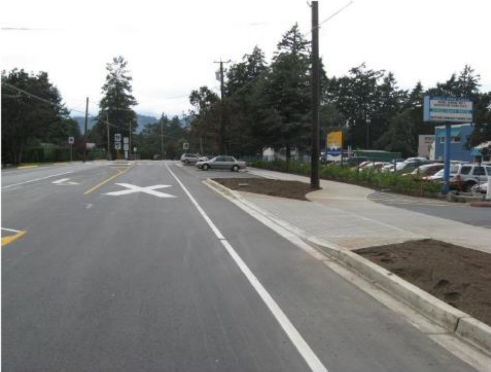
View looking west across the front of Spencer Middle School showing bicycle lane, sidewalk winding behind the parking, and properly marked turning lanes.
